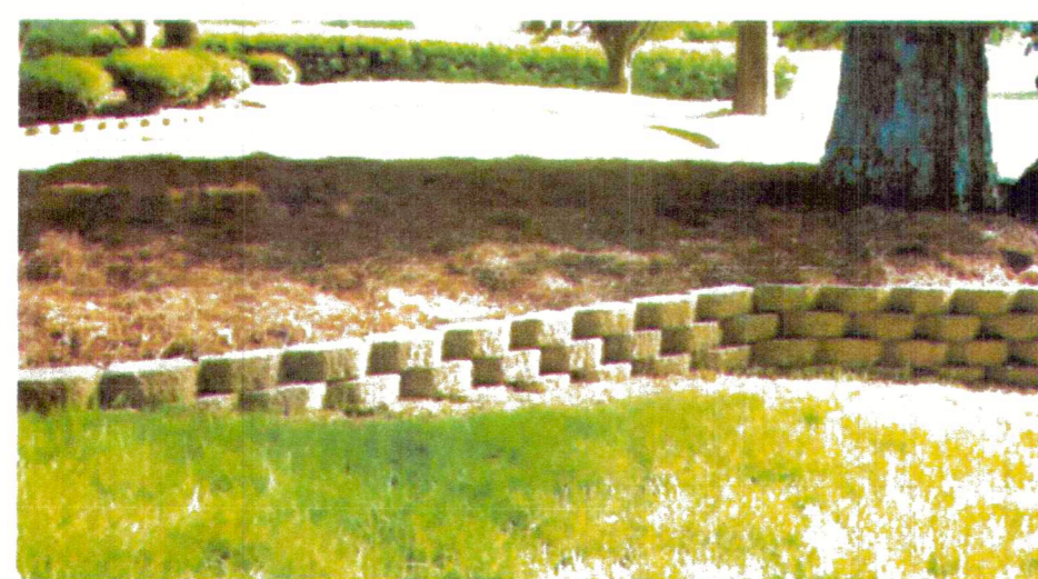
This wall is stepped up to fit the contours of the slope.
