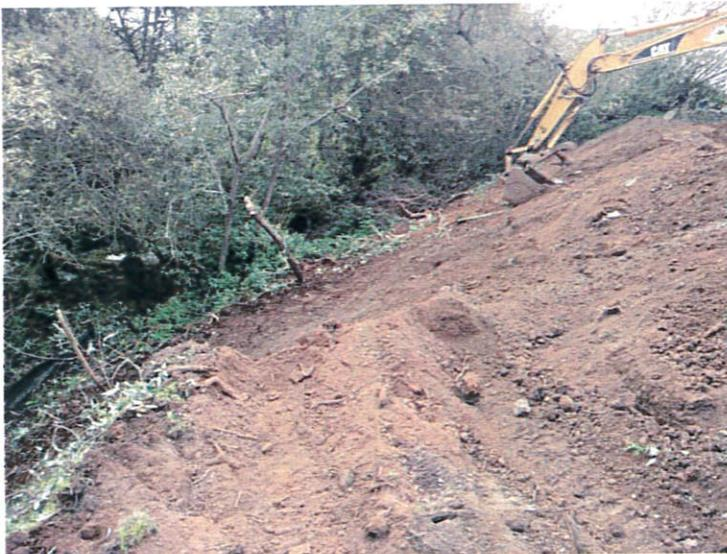
Photo 4: Excavation proceeding to toe of fill
