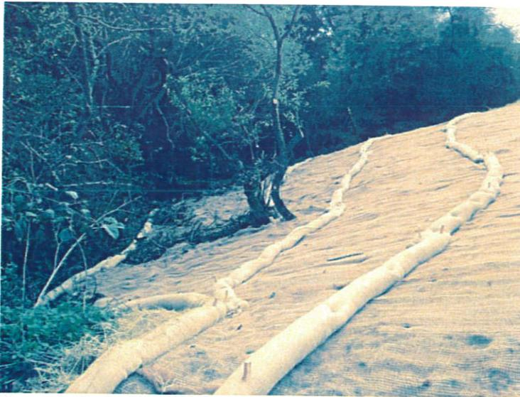
Photo 6: Final erosion control
