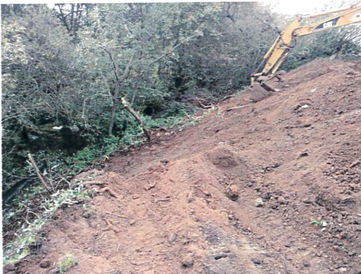
Photo 4: Excavation proceeding to toe of fill
