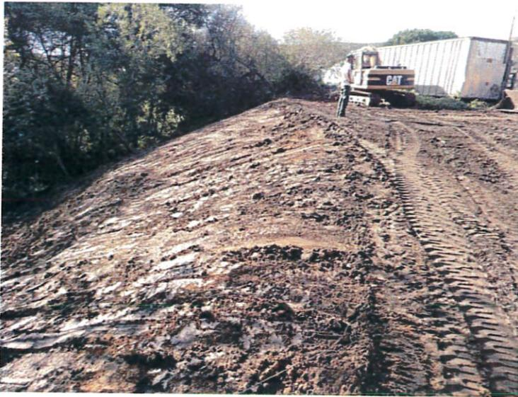
Photo 5: Final excavated slope
