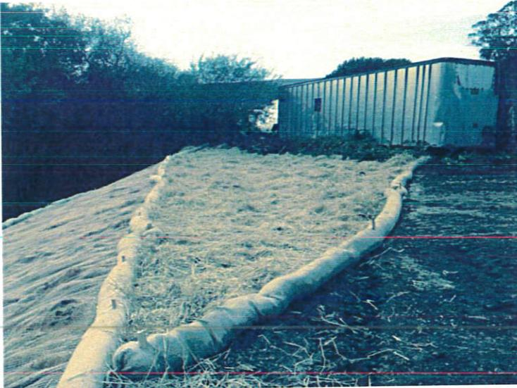
Photo 7: Final erosion control
