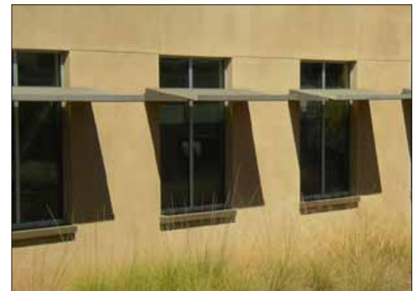
Vertical and horizontal shading elements
