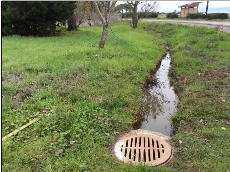
Photo 6. Stormwater drain at eastern terminus of the ditch.
