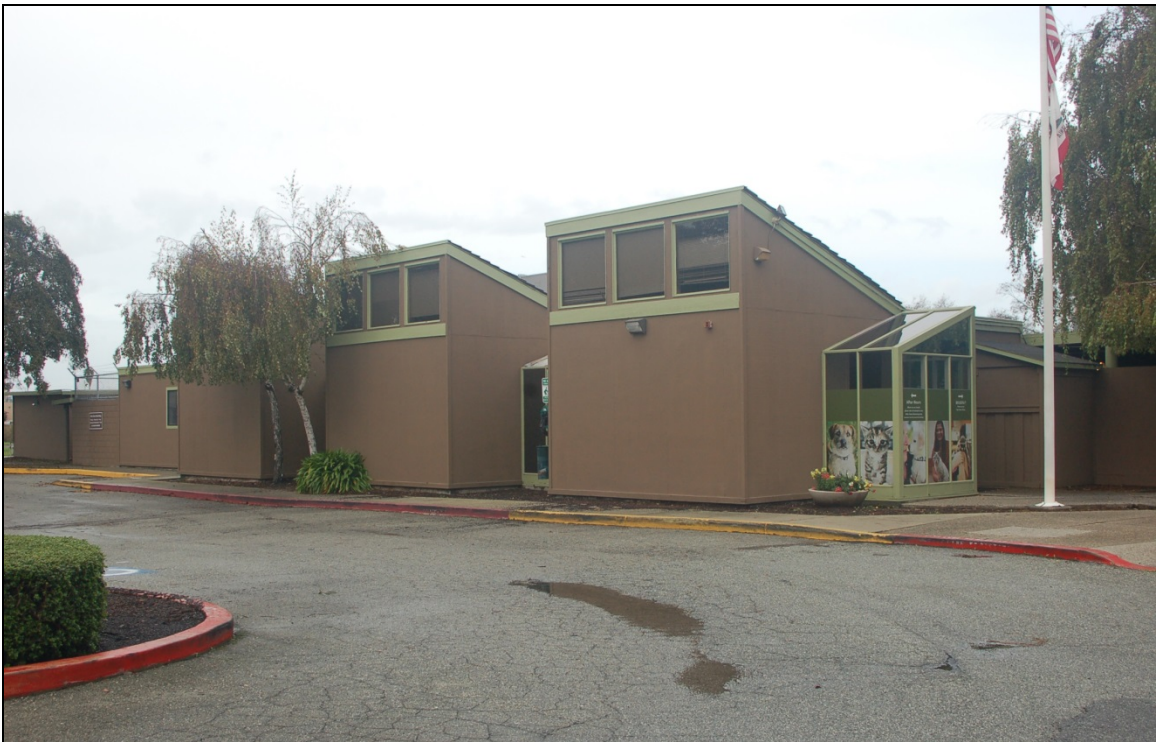
South façade of 1985 south addition to original building – view to the northwest
