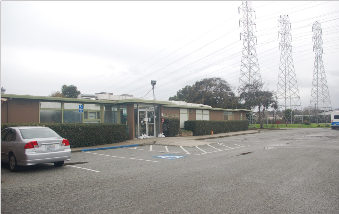
West façade of original building (current spay clinic) with projecting entrance bay - view to the southeast
