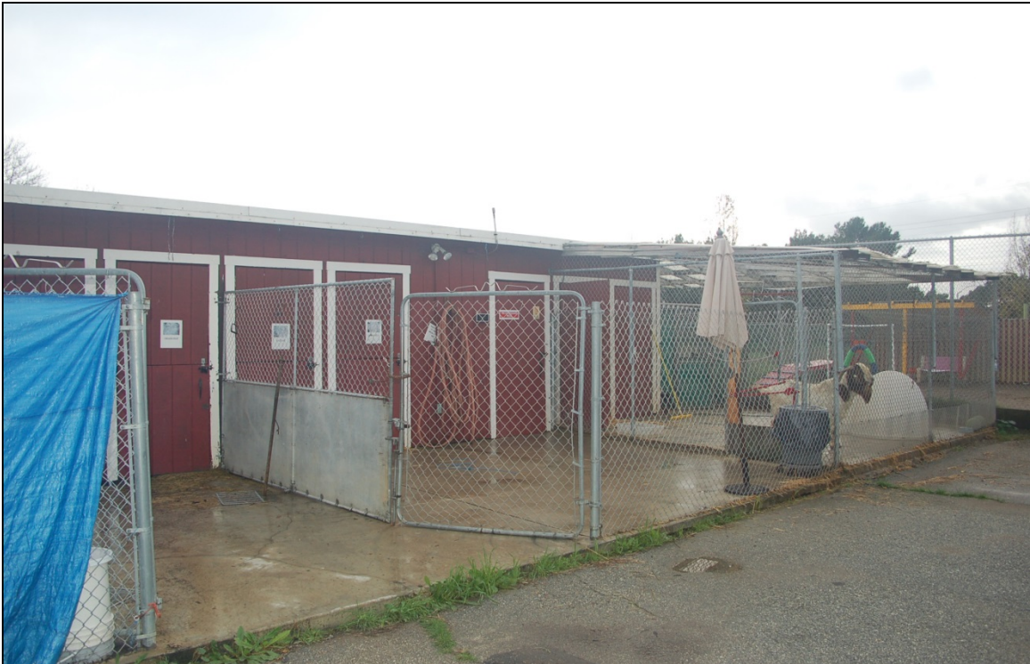
Main outdoor kennel area to the west of the central public lobby area
