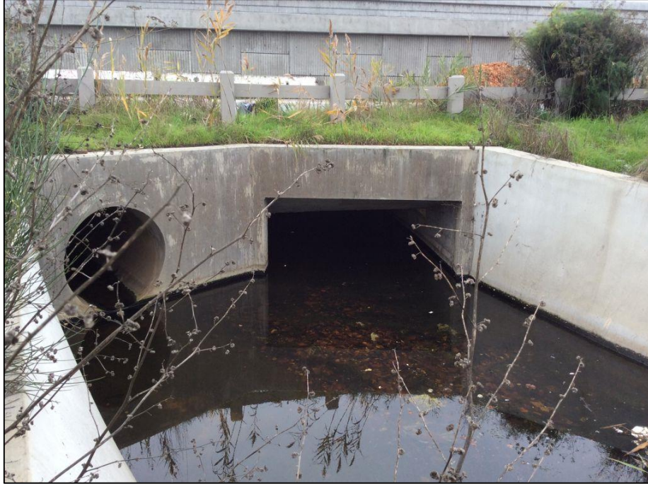
Photo 5. Perennial stream habitat (OW1).
