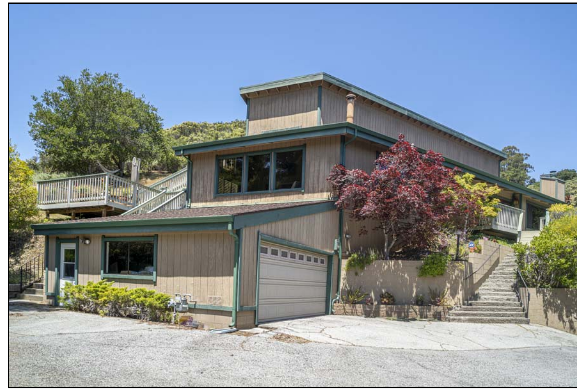
existing view at street
