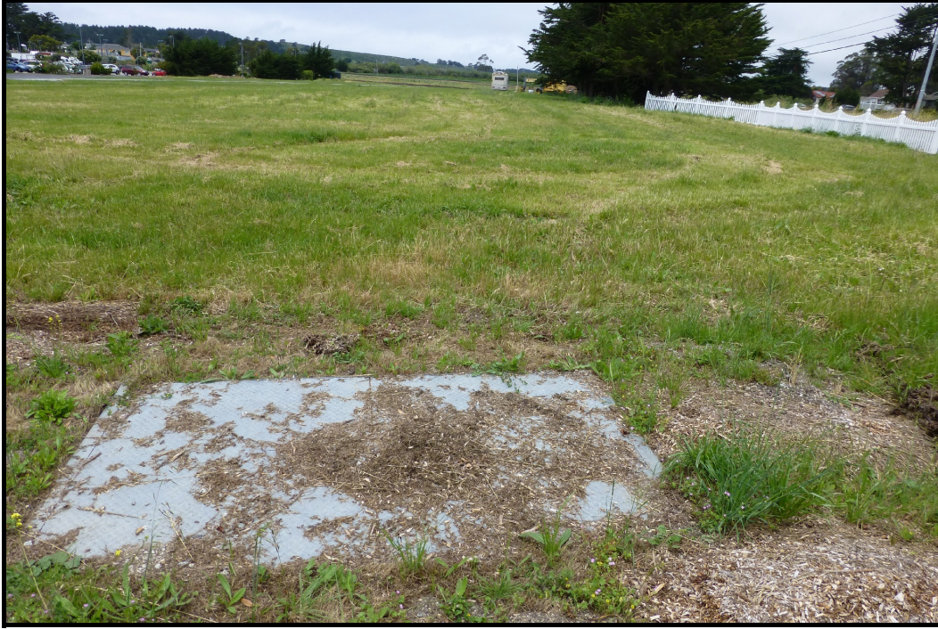
Figure 1: Harbor Village RV Park Project Area, looking northwest from south-central property fence, Highway 1 to right, buried utility box in foreground (02 June 2019).
